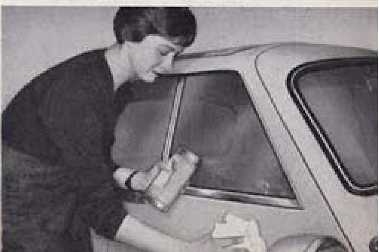
The finish is well treated when water being poured upon it is repelled in beads. The product "BMW Hard-gloss Polish" is applied with a soft polishing cloth or polishing cotton, in small quantities upon the completely dry finish, doing only a small area at a time. Next dry the body and then rub it down, using a clean polishing cloth, until original brilliance is restored.
